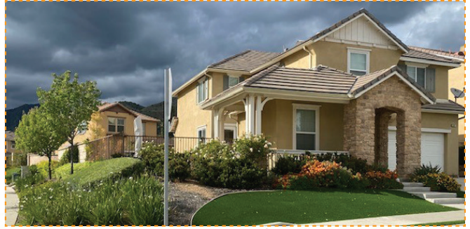
This home provides a good example of defensible space.
